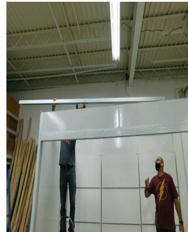
Attach Aluminum Channel to top of Front wall.
