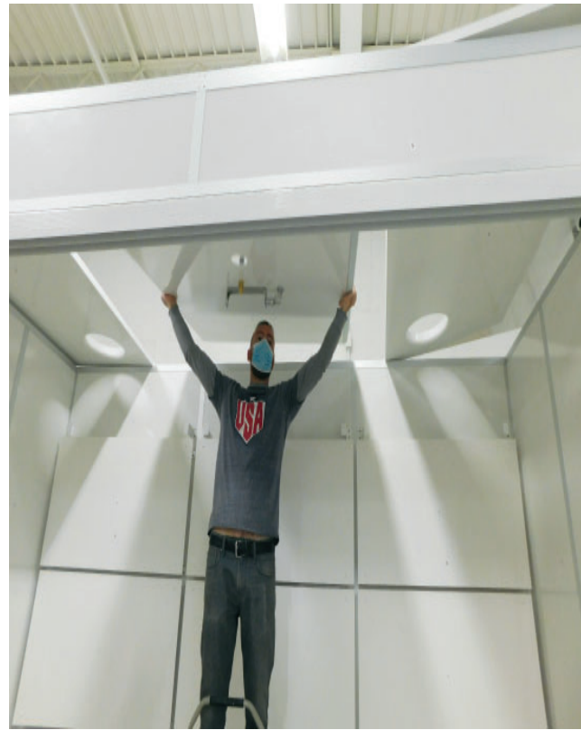
Install (Ceiling Panel C) into Aluminum channels.
