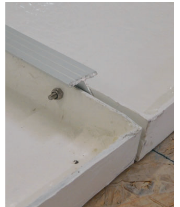
Aluminum channel shown in position between ceiling panels.
