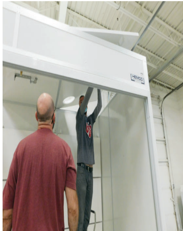
Install (Right Ceiling Panel D) into Aluminum channels.
