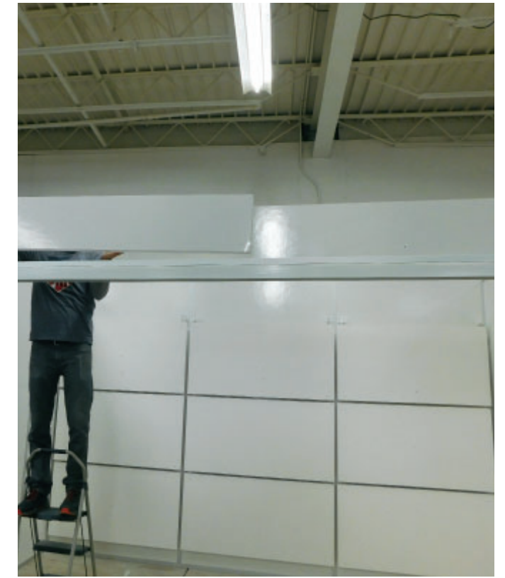
Attach (Left Header F) to top of Front wall.
