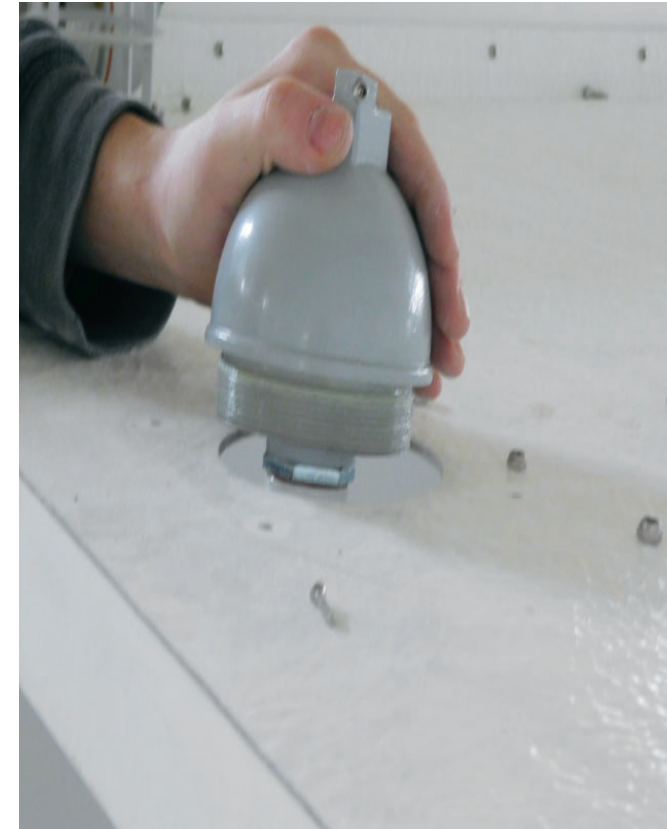
Install Top Section of Light fixture trough roof of ceiling panel
