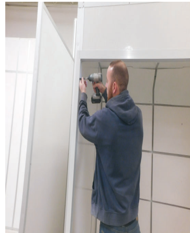
Install (Sliding Door Frame) into (Steel Door Frame)..
